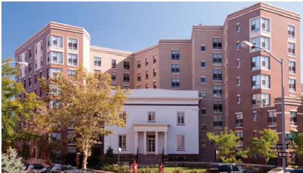
VIEW FROM EAST 156TH STREET AND BECK STREET
